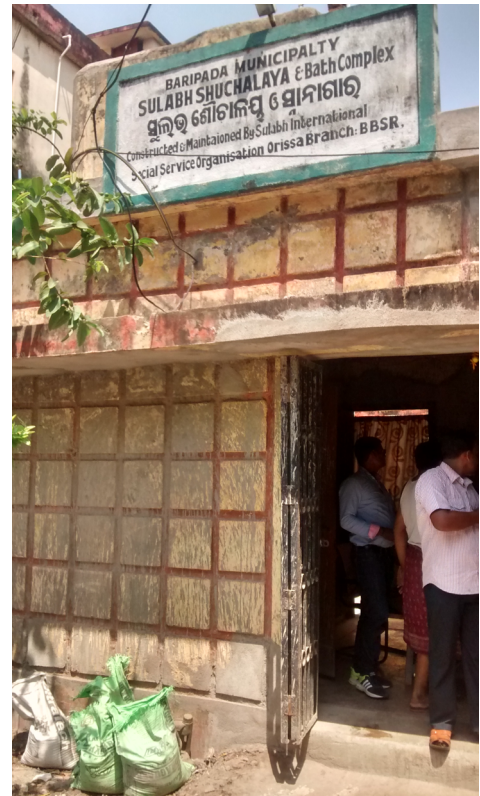
Figure 6: Public Toilet in Baripada
